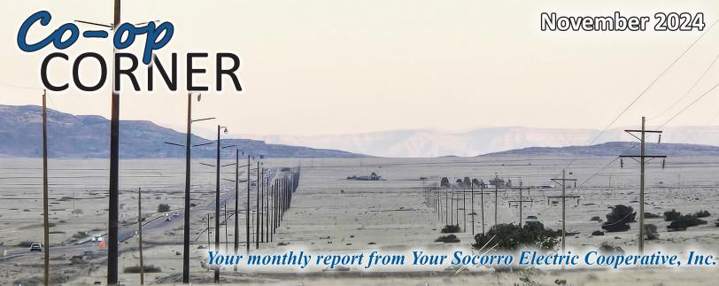
SEC's new Socorro to Magdalena 69 kV line construction showing the old transmission line on the right, the new one on the left and the distribution lines next to the new line, that will all be incorporated and moved onto the new steel poles. Photo Credit: Jimmy Capps
